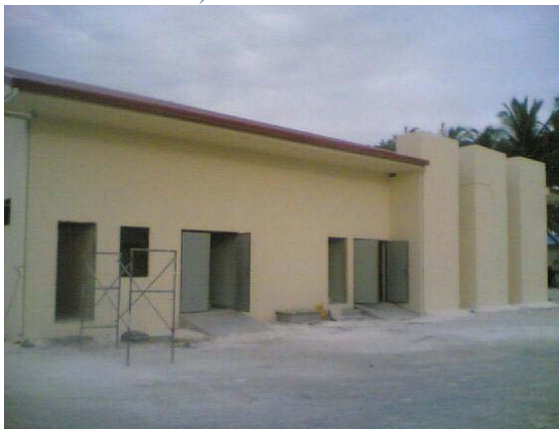
FIGURE 7: New Powerhouses Constructed under the Project, (Source: MEEW/OIEP)
