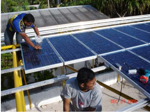
FIGURE 11: Installation of Solar-Diesel Hybrid System in Adh. Mandhoo (12kWp)
