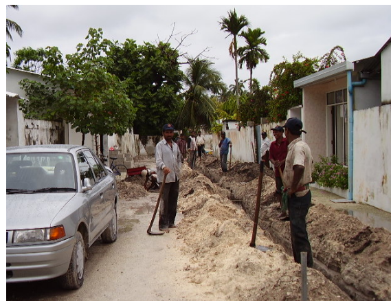
FIGURE 6: Excavation of Trenches for Laying New Distribution Network, (Source: MEEW/OIEP)
