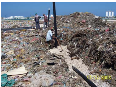
FIGURE 17: Landfill gas recovery plant construction
