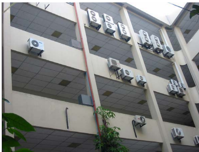
FIGURE 24: Air condition load contributes to the peak demand in Male’ (Source: SMILES Project).
