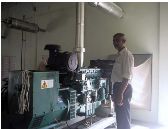
FIGURE 5: New Generator Sets Installed under the Project, (Source: MEEW/OIEP)
