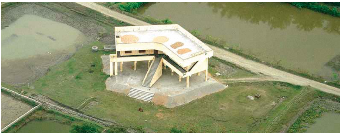
Photo: A multi-purpose cyclone shelter
